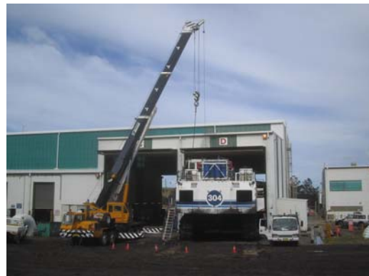
A 50 tonne crane set up to remove the engine from an excavator.
